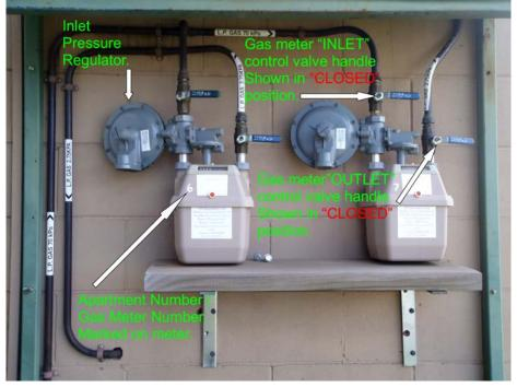
Gas meter control valve in open position: When handle is in line with pipe it is OPEN.
